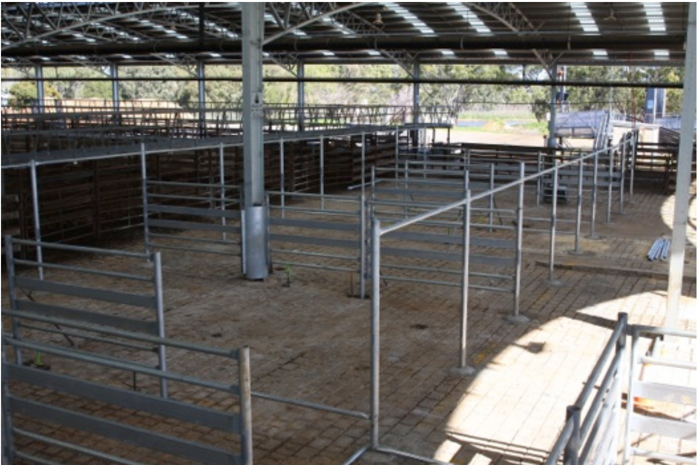
Yards under construction as part of the loading ramps project
