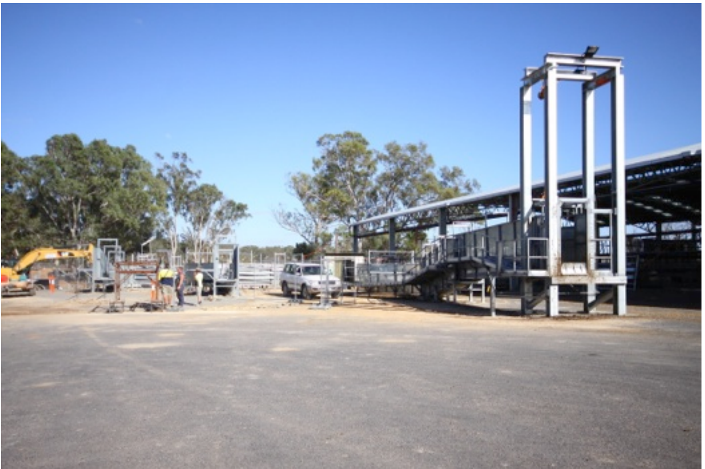
Cattle loading ramps under construction
